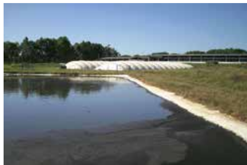
Figure 10. A manure treatment plant
