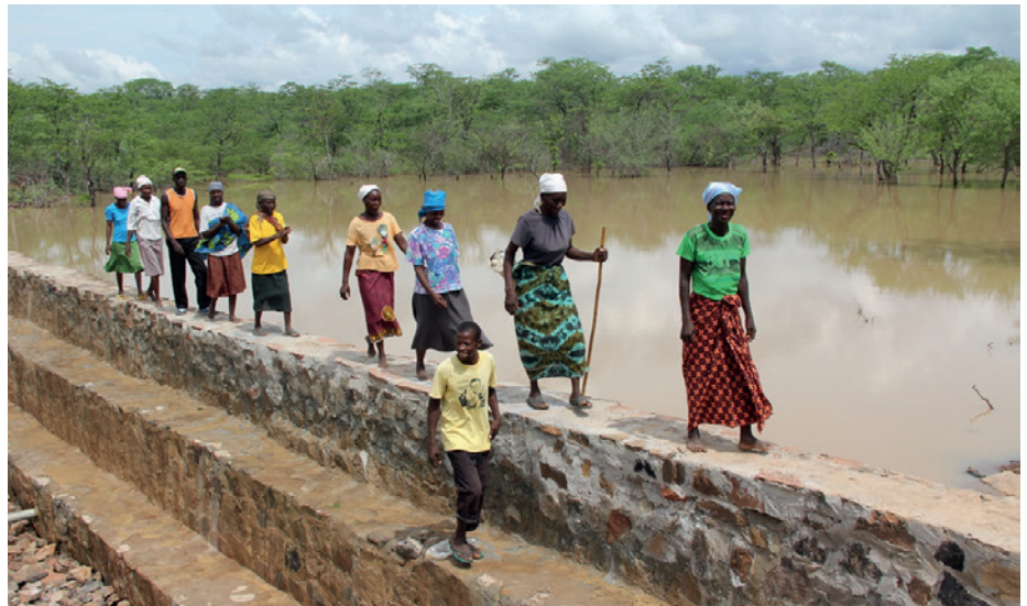
Zimbabwe - Chininga dam was constructed under the WFP-funded Food-for-Assets and resilience building programme. Photo: UN/Sirak Gebrehiwot
